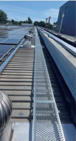
Steel Rooftop Walkway
